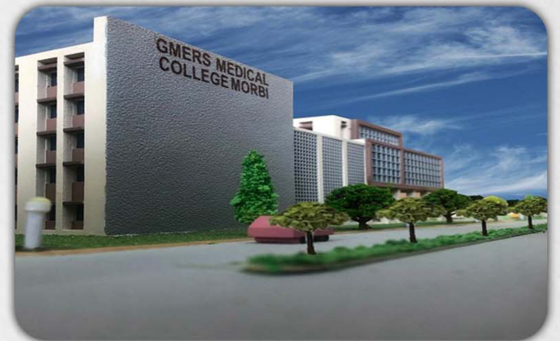
Renovation Work at CIVIL Hospital and GMERS College at Morbi.
