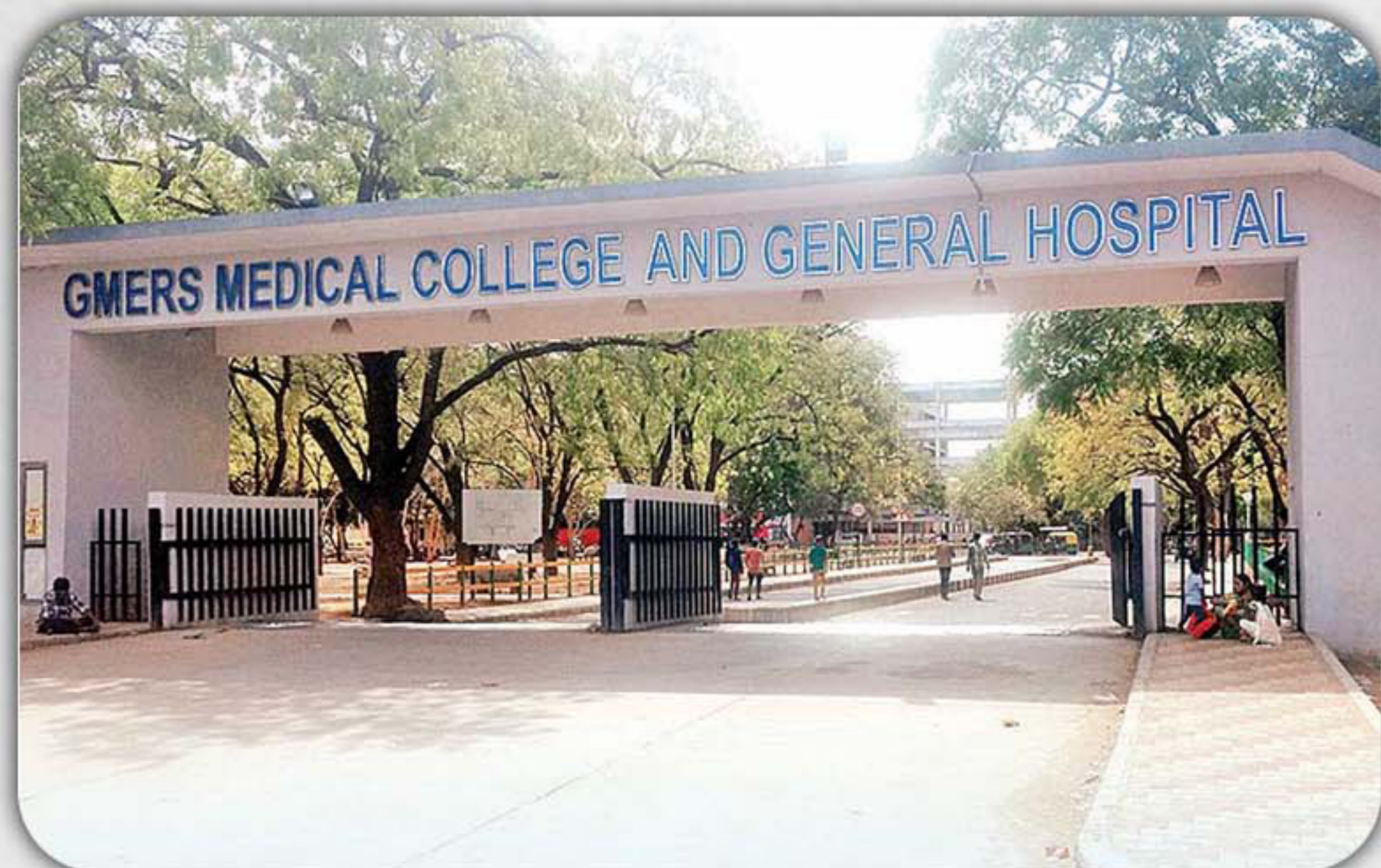
Super Speciality Hospital (Annex Building), Critical Care Center & Rain basera as Expansion of GMERS Medical College at Gandhinagar. – Gujarat
