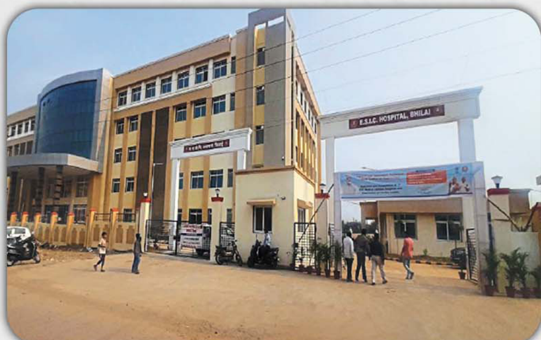
100 Bedded ESIC Hospital at Bhilai, Raipur (C.G.) Chhattisgarh
