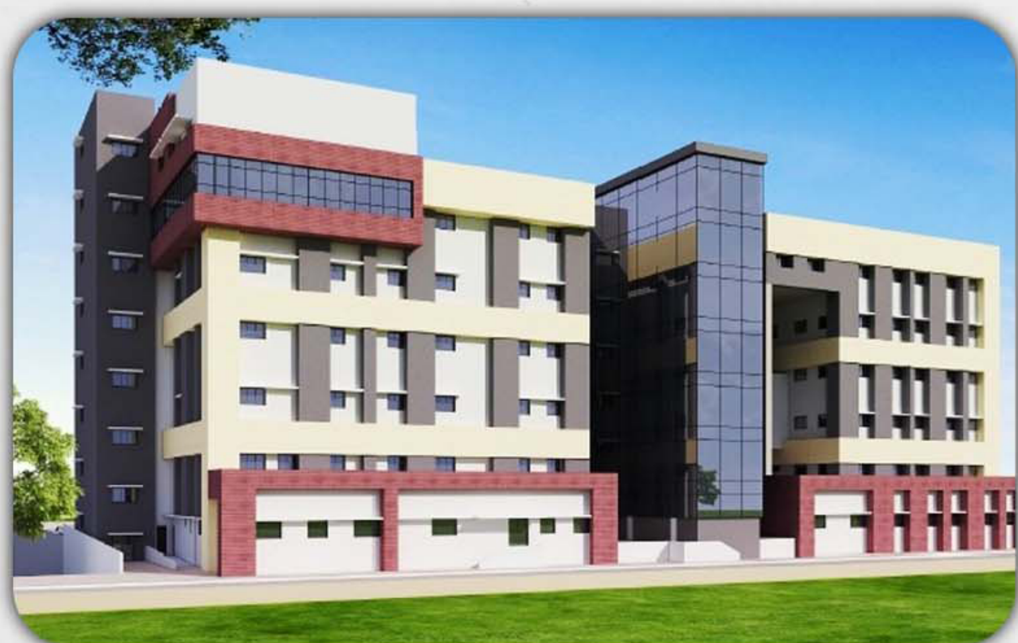
Renovation Work at PDU Hospital at Rajkot.
