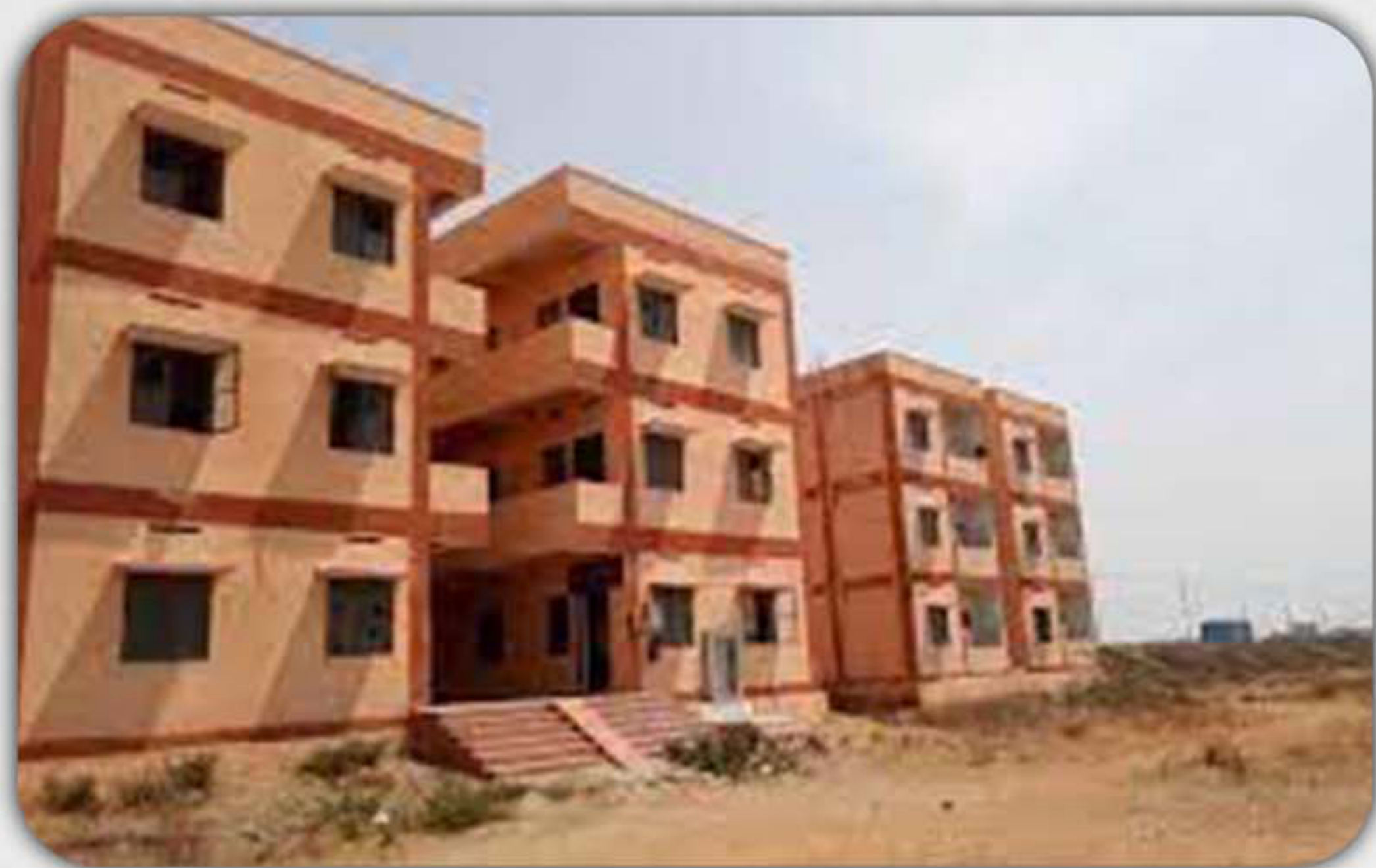
Constnution of Staff Quarters at Sudamada, Dist - Surendranagar.
