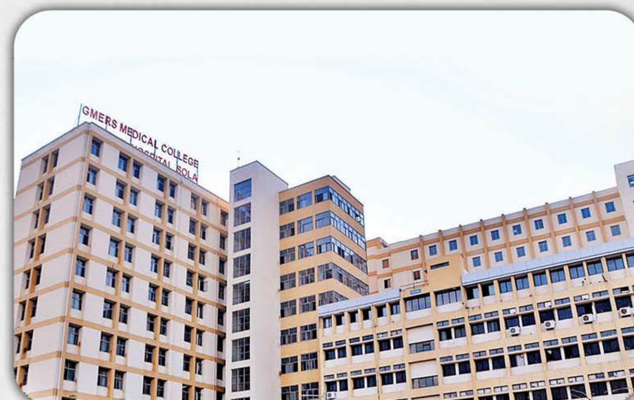
Super Speciality Hospital as Expansion of GMERS Medical College at Sola, Ahmedabad. Gujarat
