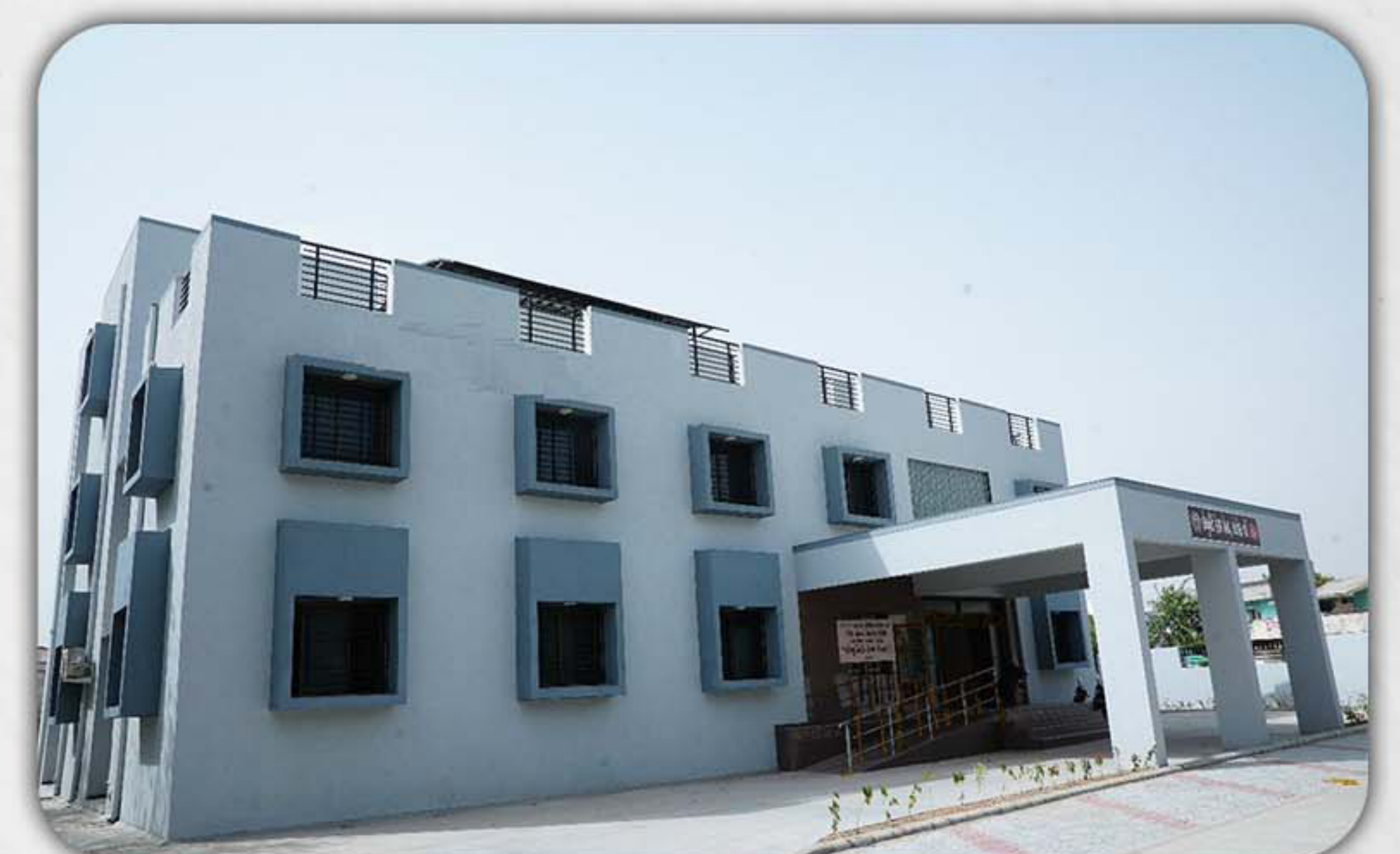
Constnution of Community Health Centre at Datha, Dist - Bhavnagar.
